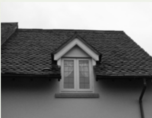
(Figure 16: mixed shingle tiled roof)
