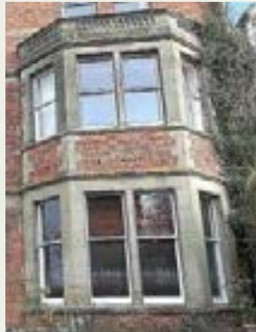
Sandstone Lintels and decoration
