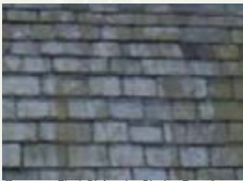
Course Flat Shingle Slate Roof
