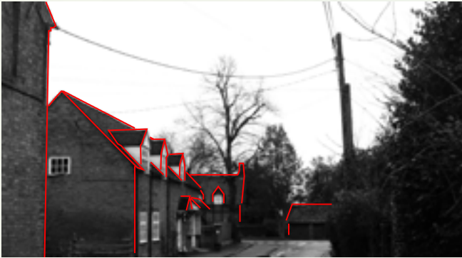
(Figure 28: Village Centre Cottage Roofscape)
